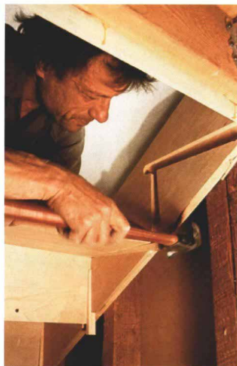
Much of the new stair is supported by housed carriages screwed to the wall framing. In the photo to the left, one of the carriages can be seen just to the left of the ladder. On the dining-room side of the second flight, the ends of the treads are exposed to view. They bear on the 2x blocks shown here as they're being installed by Ivan Rainer. In the photo above, Rainer taps home a freshly glued wedge to secure a tread on the second flight.
