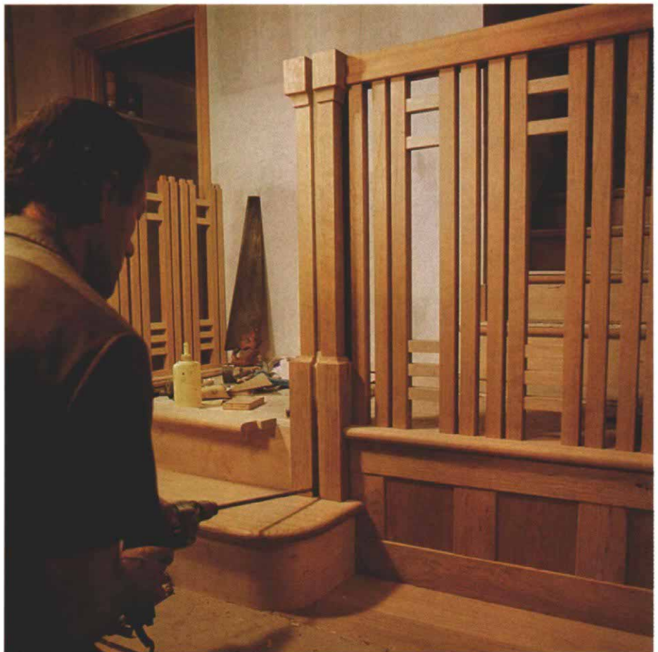
Using an electric iron, the author applies heat to moist rags as he bends a piece of \frac{3}{4} in. thick maple for a riser. The curved portion of the maple is a scant \frac{1}{8} in. thick, but it will be permanently backed by the curved block used here to anchor the clamps.
