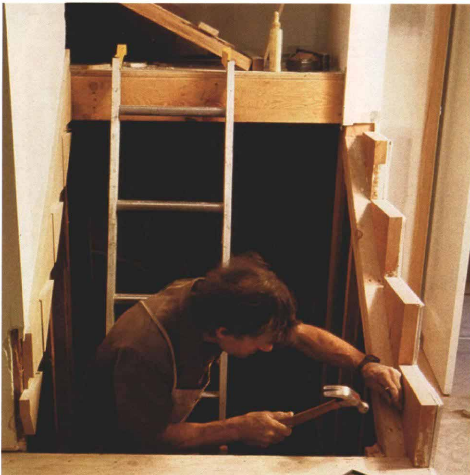
Much of the new stair is supported by housed carriages screwed to the wall framing. In the photo to the left, one of the carriages can be seen just to the left of the ladder. On the dining-room side of the second flight, the ends of the treads are exposed to view. They bear on the 2x blocks shown here as they're being installed by Ivan Rainer. In the photo above, Rainer taps home a freshly glued wedge to secure a tread on the second flight.
